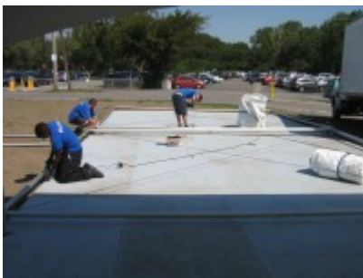
installation plancher gris
